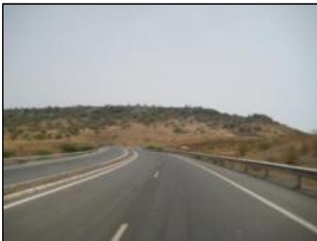
Fig.4: Praia city - Cape Verde - The new radial highway . Can
