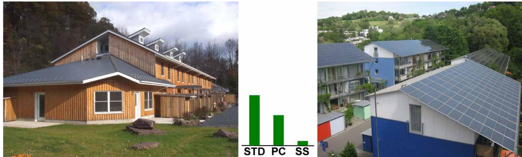
Figure 6: Comparative energy use (for heating and cooling per m 2 ) of “Green” Affordable Housing at Petersburg Commons (PC), left, and Schlierberg Solar Estate (SS), right.
